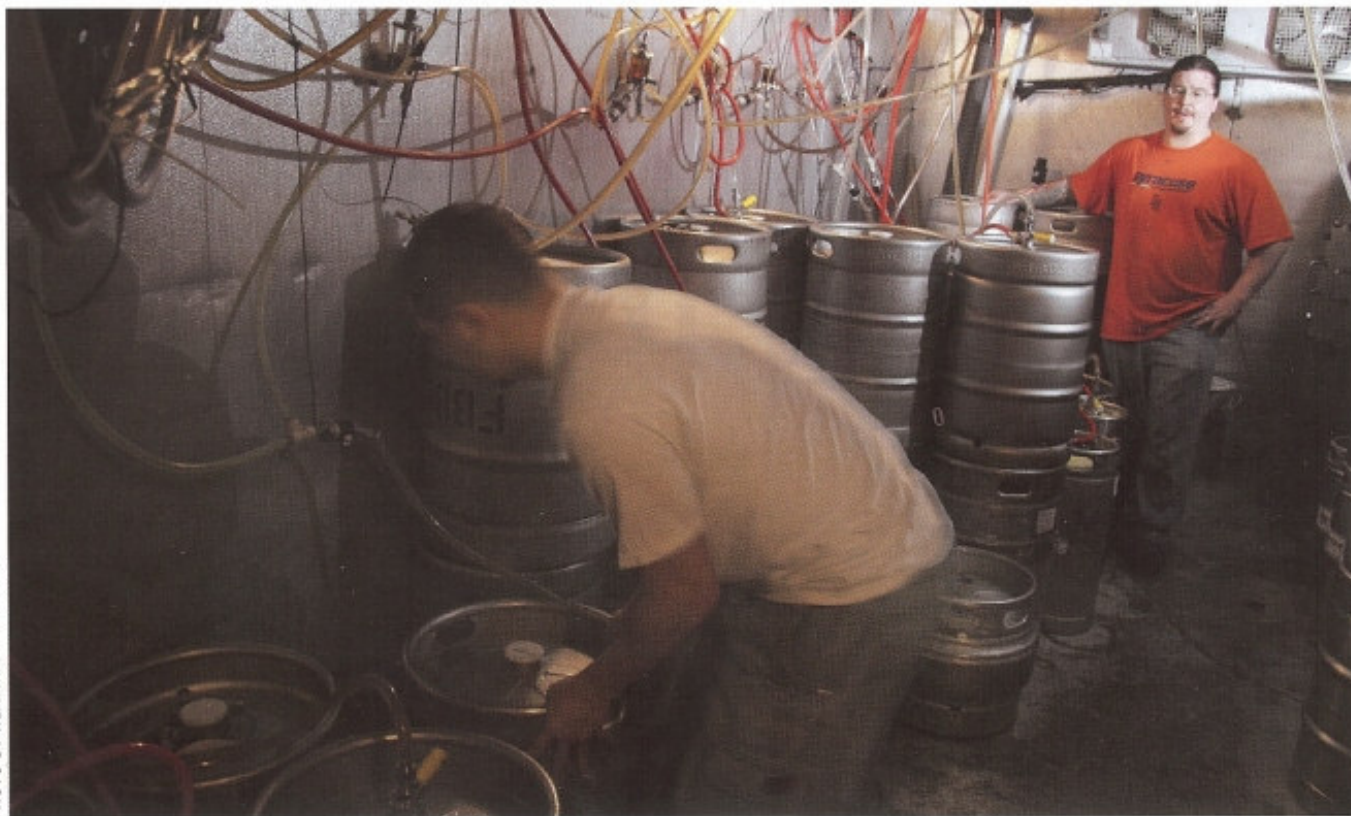
Empire Brewing Co.'s Brewmaster Tim Butler oversees his assistant Dan Martin hooking a keg of beer to the tap. US Beverage Net installs one flow meter per beer line in the keg storage room and then is connected to a data transmitter, sending information to a secure Web server. The company easily can review and compare revenue against actual product movement in real time.
